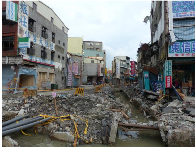
Fig. 3. Street affected in the Kaohsiung explosion (photo by Syuan Shih Sheng)
